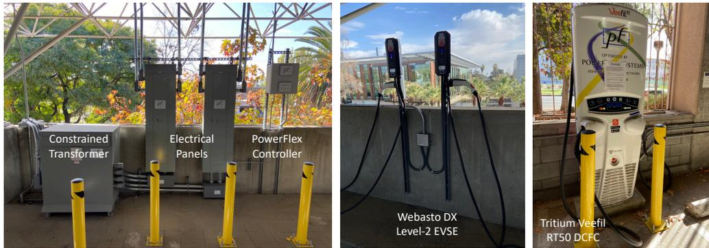
Figure 3.1: Photos of the N\_Wilson\_Garage\_01 ACN, which is one of the charging sites used to collect data.
