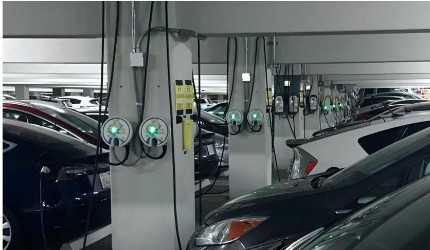
Figure 1.4: The ACN smart EV charging testbed at Caltech.
