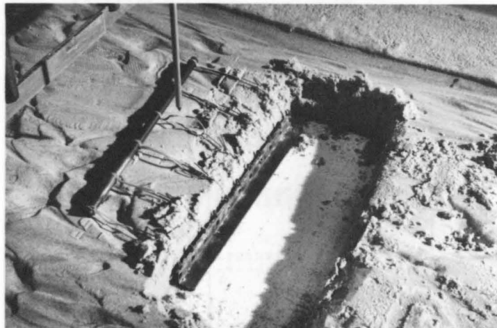
(b) Installation in flume showing pre-burial support hooks.
