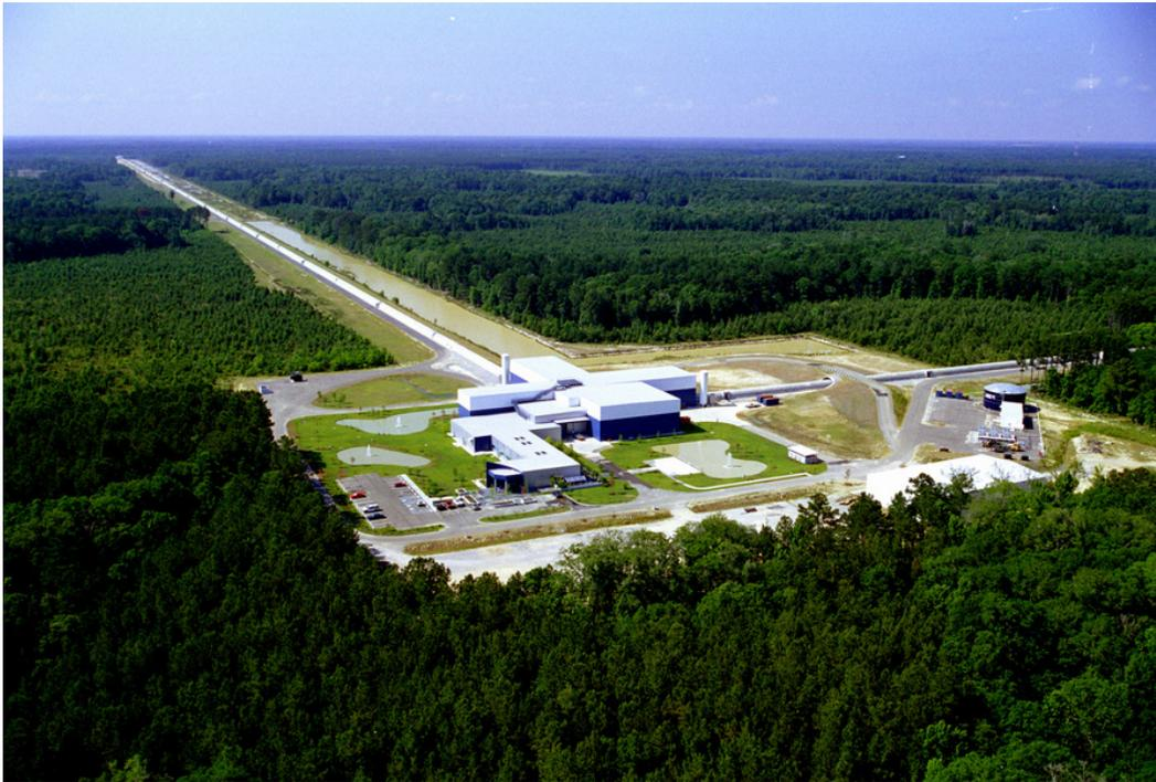
Figure 1.3: The LIGO Laboratory operates two detector sites, one near Hanford in eastern Washington, and another near Livingston, Louisiana. This photo shows the Livingston detector site. Credit: Caltech/MIT/LIGO Lab.
