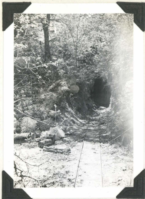
A. TUNNEL PORTAL, HIMALAYA LODGE, MESA GRANDE
