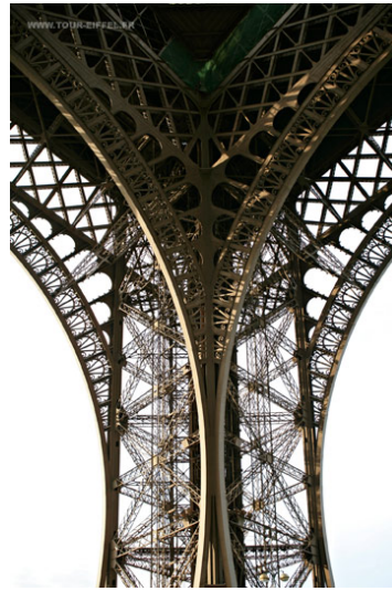
(b) Interior view of a tower leg showing trusses made of trusses. Image courtesy of B. Michau.
