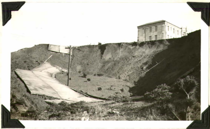
Fig. 11. Escarpment formed by landslide at its upper edge. Parker Avenue slide.
