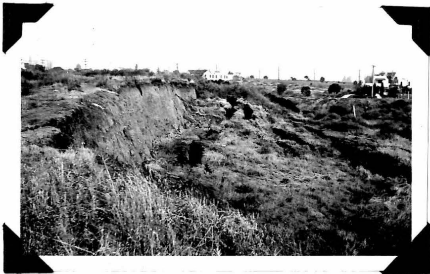
Fig. 38. Uper edge of Potrero slide showing open cracks. View looking northward.
