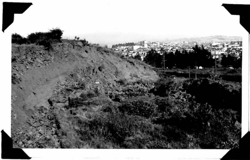
Fig. 29. Escarpment along upper edge of landslide B.
