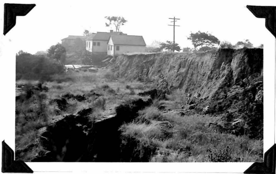
Fig. 36. Upper edge of Potrero landslide. View looking southward.
