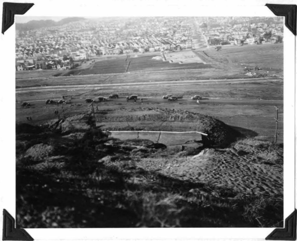
Fig. 14. Upthrust mound at the foot of Parker Avenue landslide. View looking westward.
