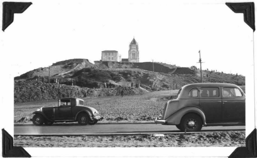
Fig. 12. View of Parker Avenue landslide looking eastward.
